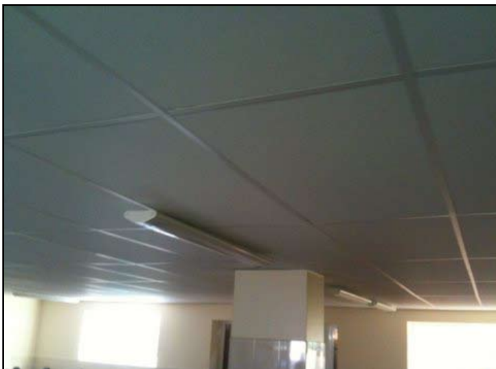
Dining Hall ceiling in Alabama Building.
