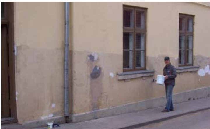
Christian friend of Edgars who is repairing the facade.
