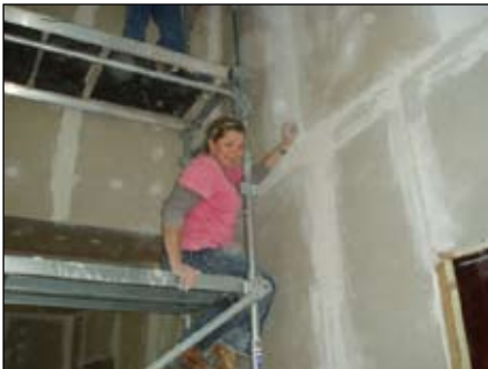
Sanding sheetrock walls
